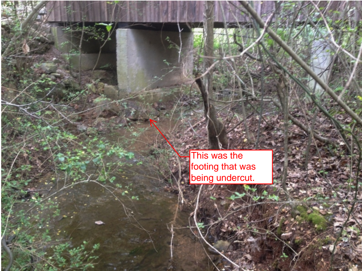
Ole 97 Bridge, a look from upstream, after work was complete. Removed a lot of the under brush to encourage erosion of the creek bank on the right side.
