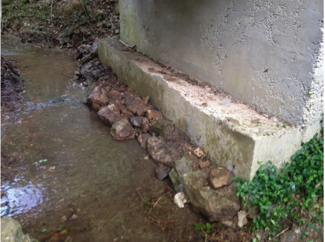
A look from the backside (downstream).
